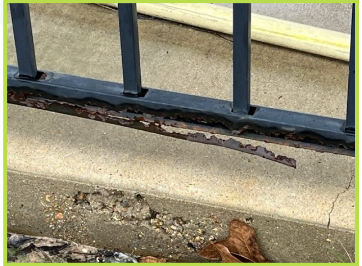
Bottom railing of fencing is rusted throughout
