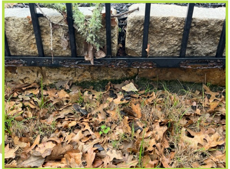
Bottom railing of fencing is rusted throughout
